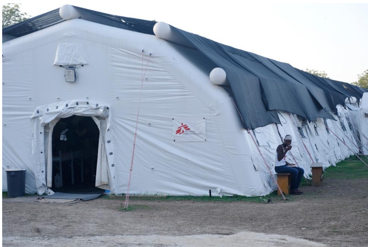
Figure 10. An inflatable structure used by Medecins Sans Frontieres for a hospital after an earthquake in Haiti. Image credit www.doctorswithoutborders.org
